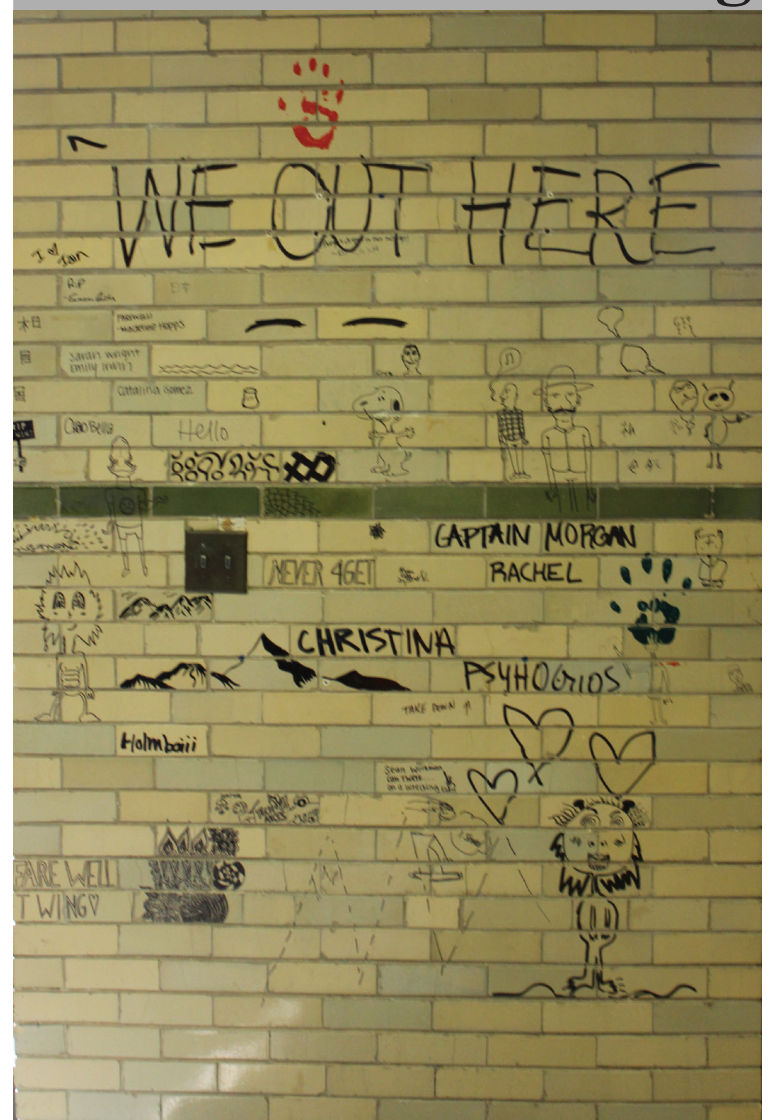
Some of the art created on Friday, Mar. 27 in the T-wing of the Winnetka Campus. Students were allowed to enter the wing and draw on the walls and windows just before demolition on the T-wing began as a part of the renovation of the Winnetka campus. For more pictures of the art, go to newtriernews.org | Clarke
