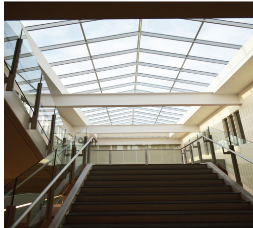
Skylight provides natural light | Zervas
