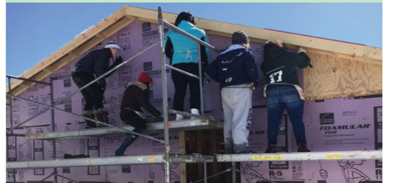
New Trier seniors help in building a house for Habitat for Humanity | Pettas
