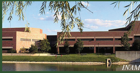
Stop undermining Oakton
